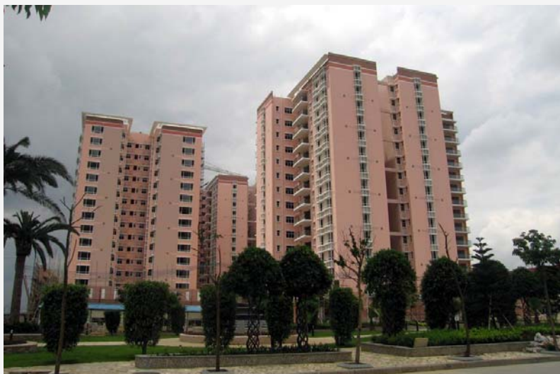
Residential Apartment (Phase 1A)
