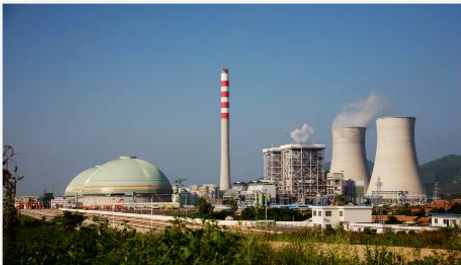
Heyuan Power Plant
