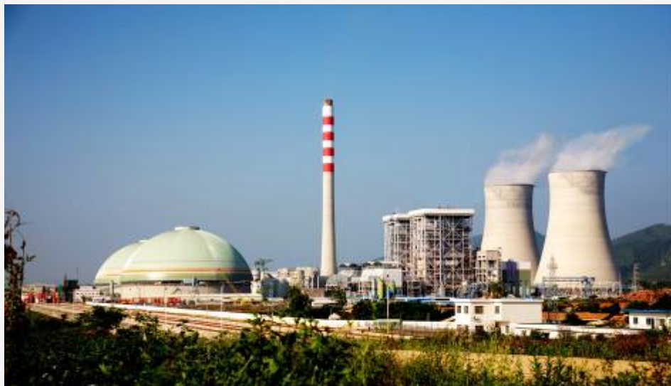
Heyuan Power Plant
