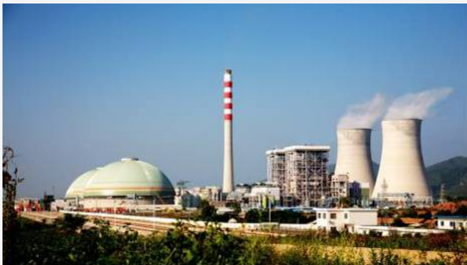
Heyuan Power Plant
