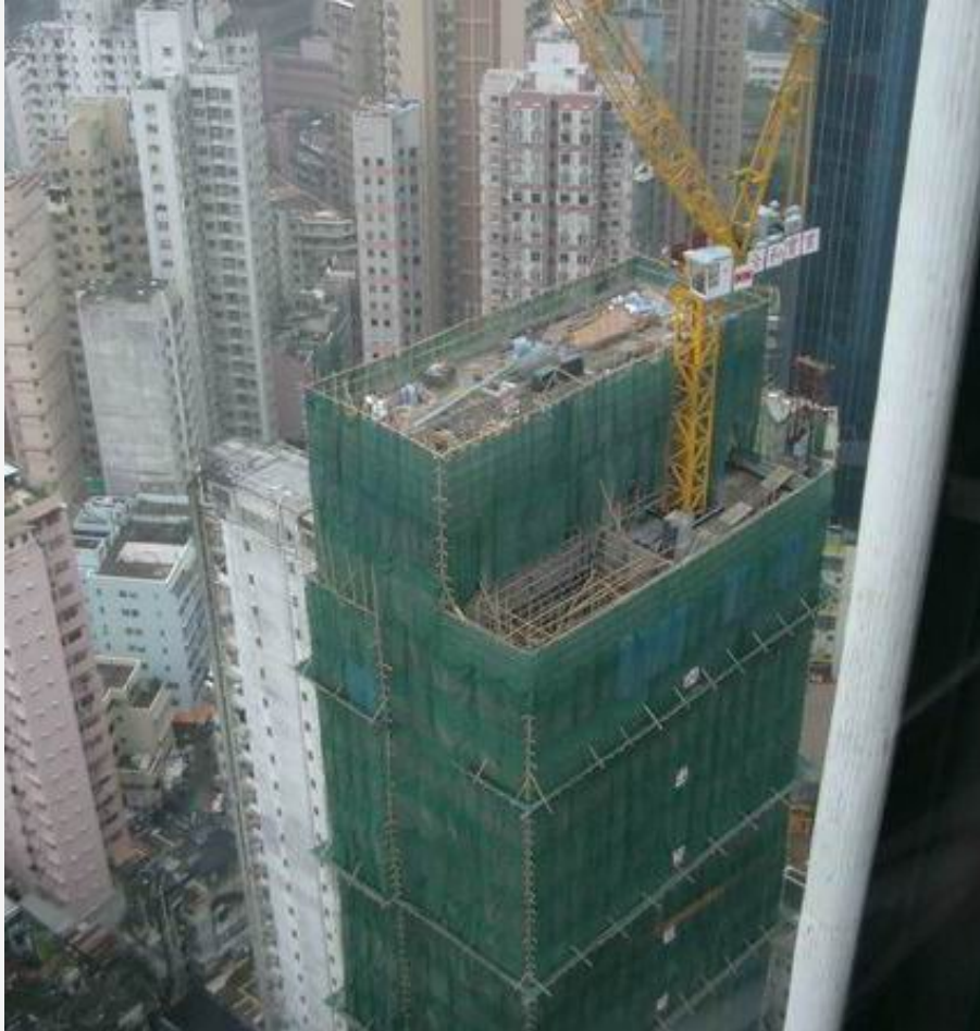
QRE Plaza under construction
