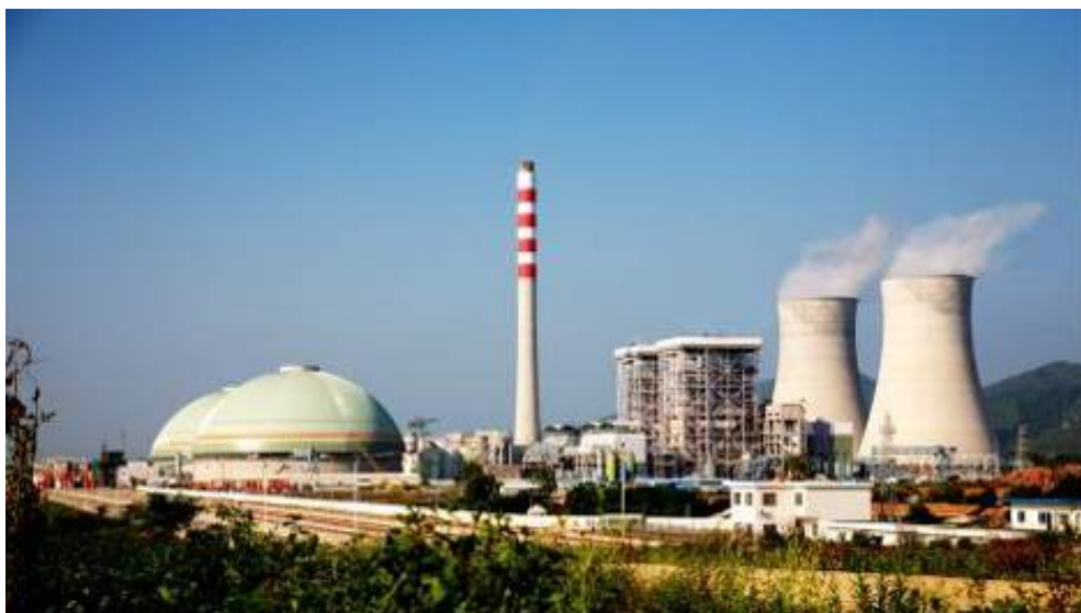
Heyuan Power Plant
