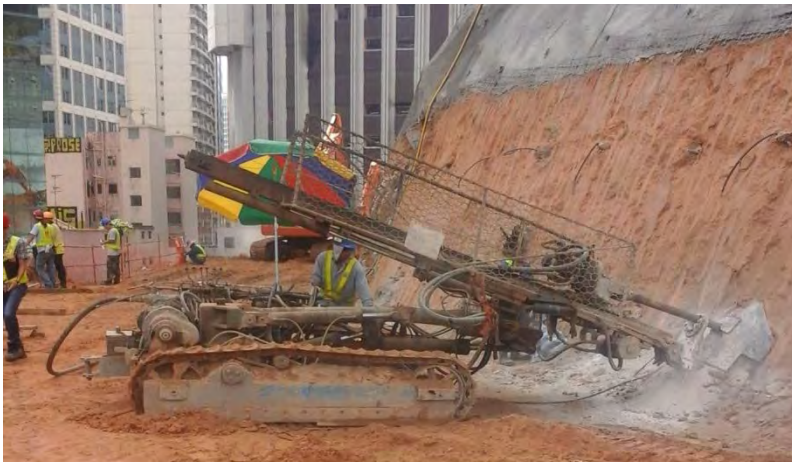
Soil Nail Installation
