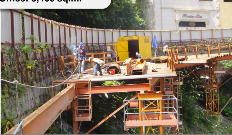
Construction of Temporary Steel Work Platform
