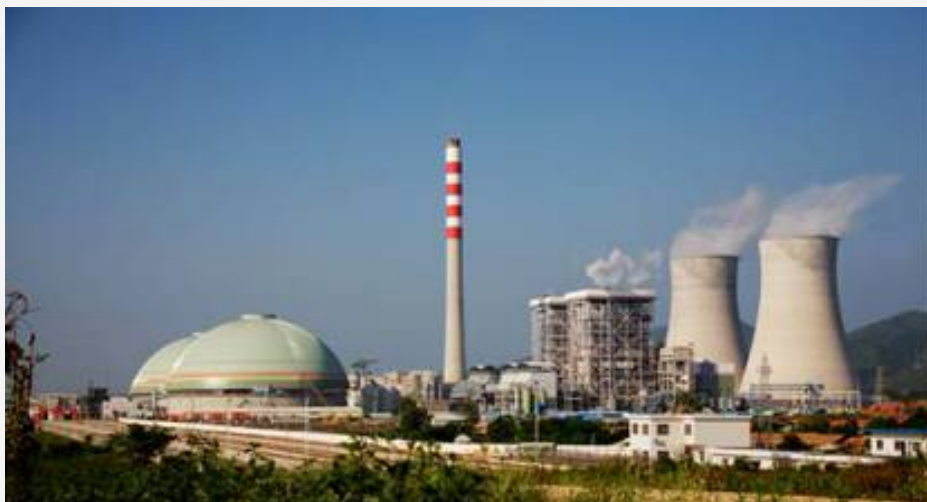
Heyuan Power Plant
