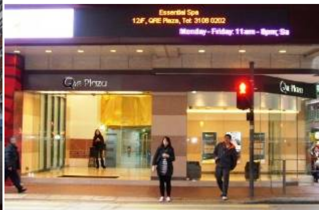
QRE Plaza main entrance lobby
