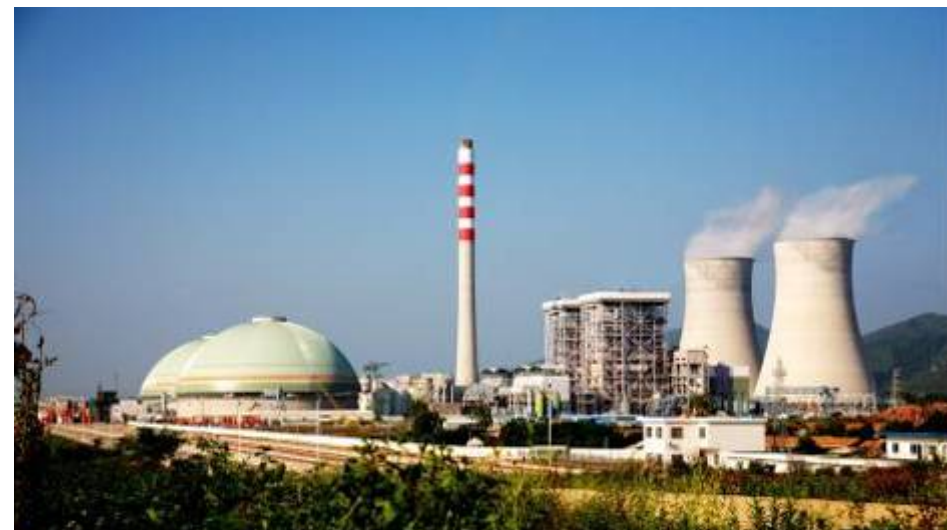
Heyuan Power Plant
