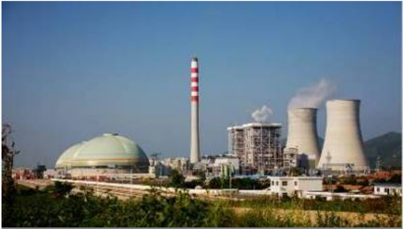
Heyuan Power Plant
