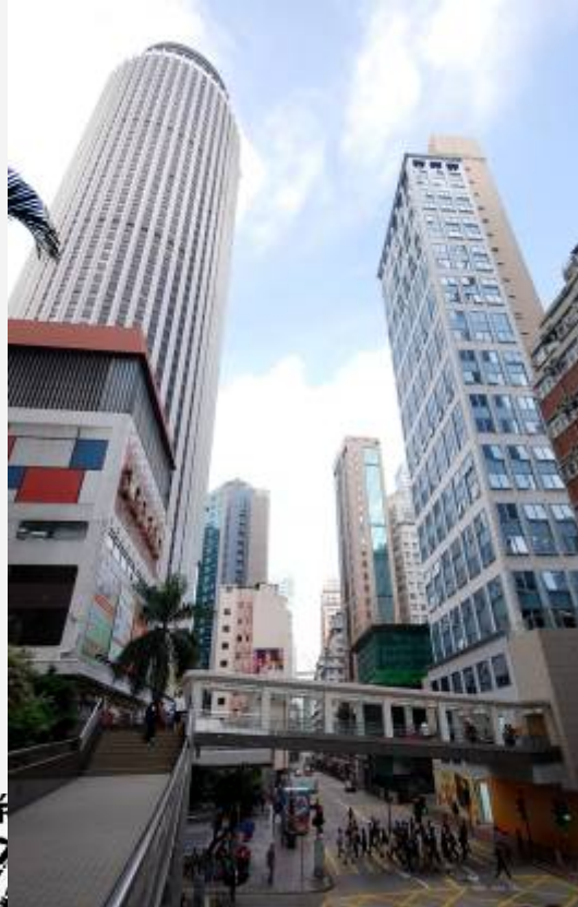
Footbridge linking QRE Plaza, Hopewell Centre and Wu Chung House
