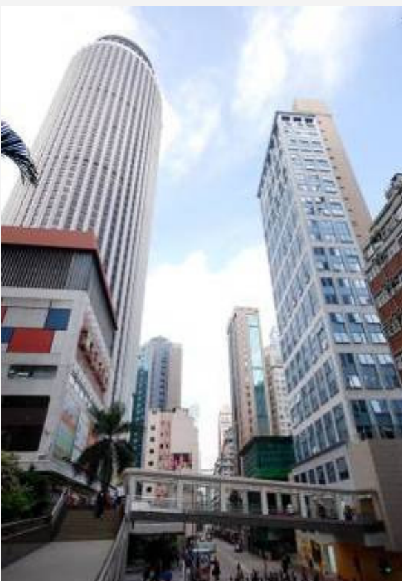
Footbridge linking QRE Plaza, Hopewell Centre and Wu Chung House
