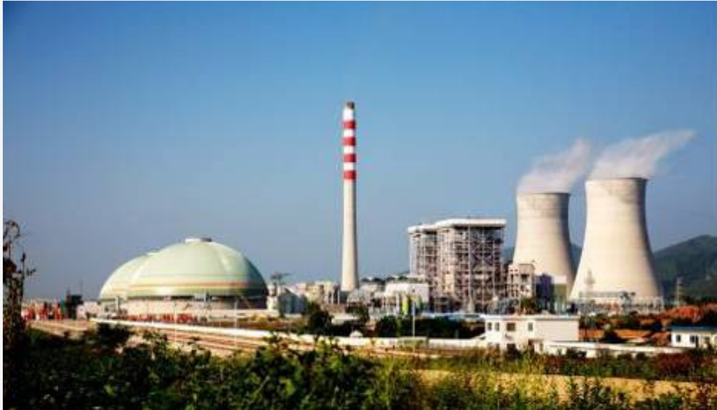
Heyuan Power Plant
