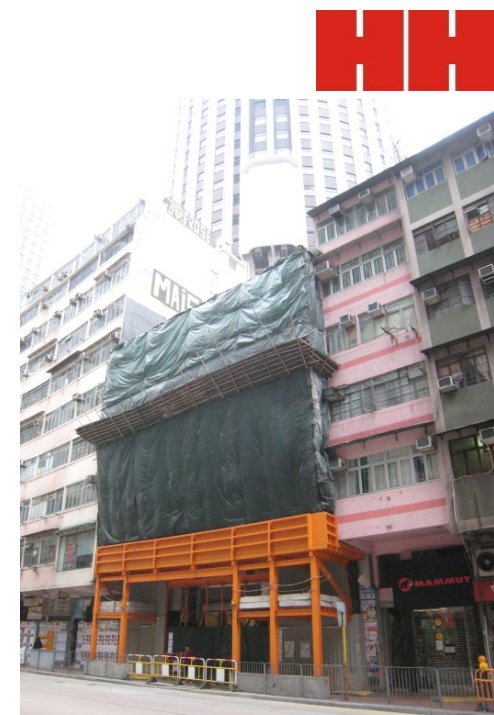
155-159 Queen's Road East – Demolition
