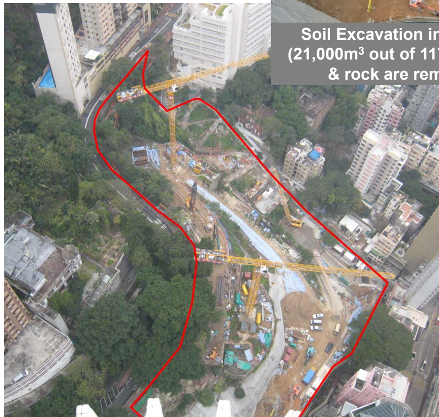
HCI Site – Site formation work in progress
