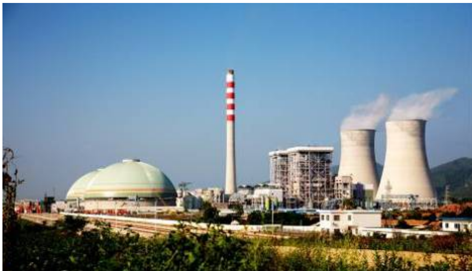
Heyuan Power Plant
