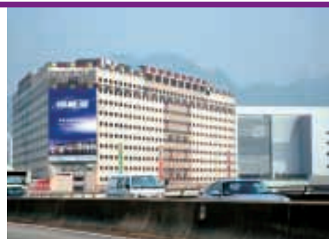
HITEC with EMSD headquarters in background
